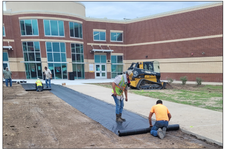
Installing the weed barrier. Photo by Jaime Flores.
