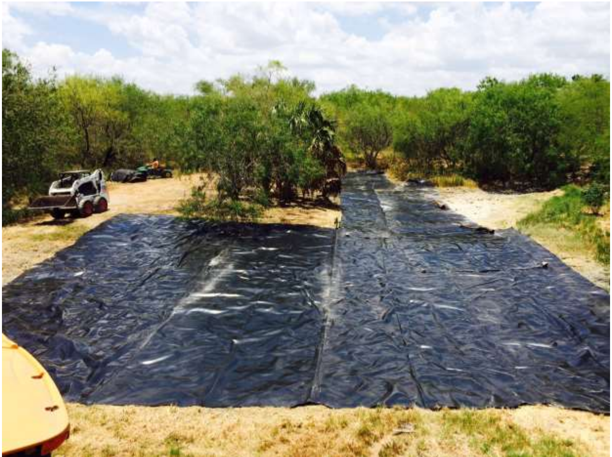
Installing liner in Pond # 4
