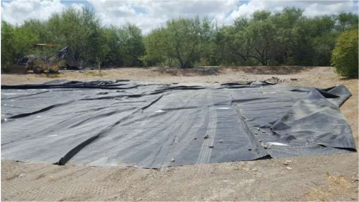
Installing liner in Pond # 3
