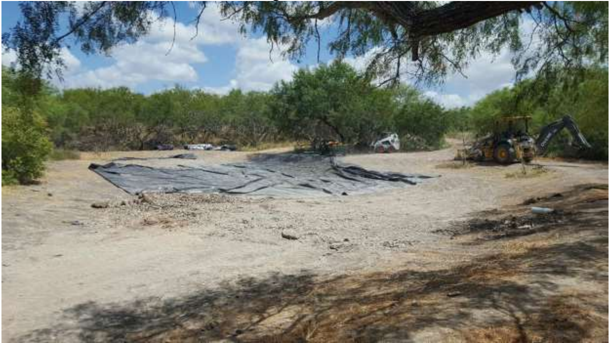
Installing liner in Pond # 3
