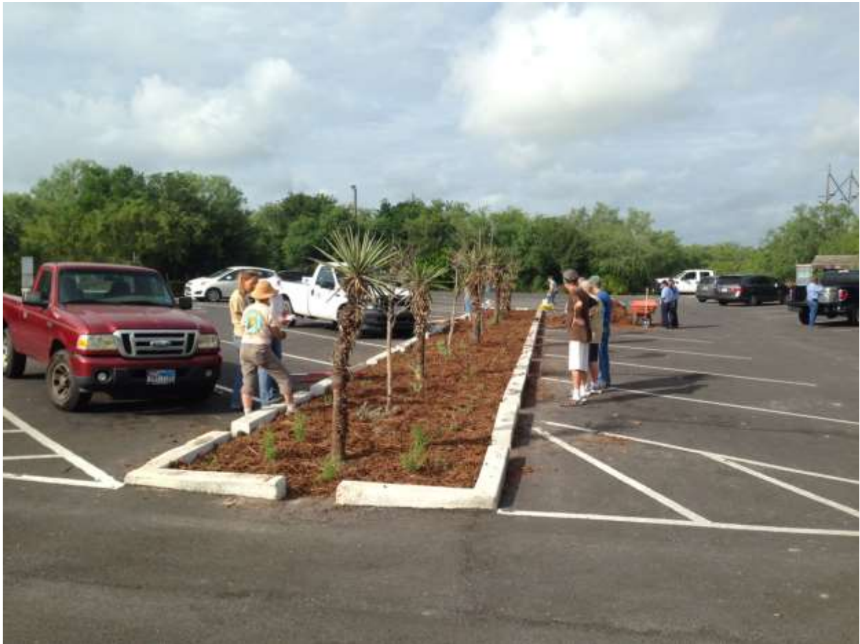
Planting of the Bio-retention Basin complete.
