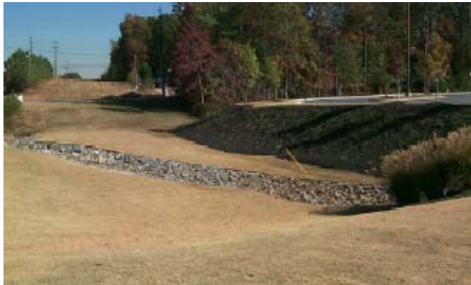
Dry Detention Basin
