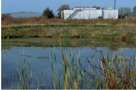
Polishing Pond with no aeration (Lopp Consulting Engineers)
