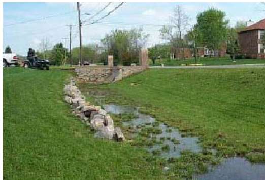
Open conveyance channel
