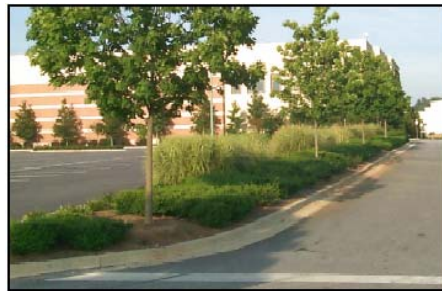
Bioretention Area ISWM Manual*
