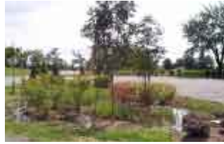
Parking lot bioretention cell day after storm. Cell designed to store water for no more than 72 hours after storm. (Massachusetts Low Impact Development Toolkit)
