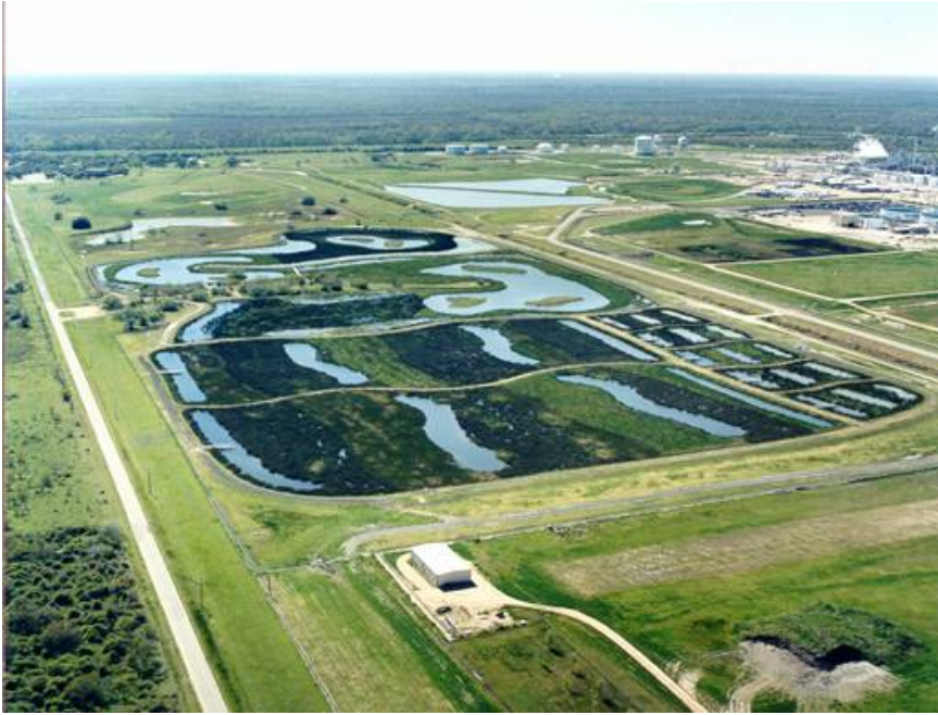
DuPont (Invista) Victoria Constructed Wetland (approximately 53 acres of wetland surface area)(Alan Plummer Associates Inc.)
