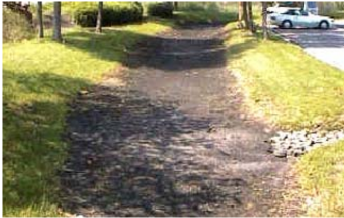
Infiltration Trench ISWM Manual
