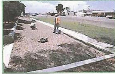
Infiltration Trench Example (Georgia Stormwater Management Manual)
