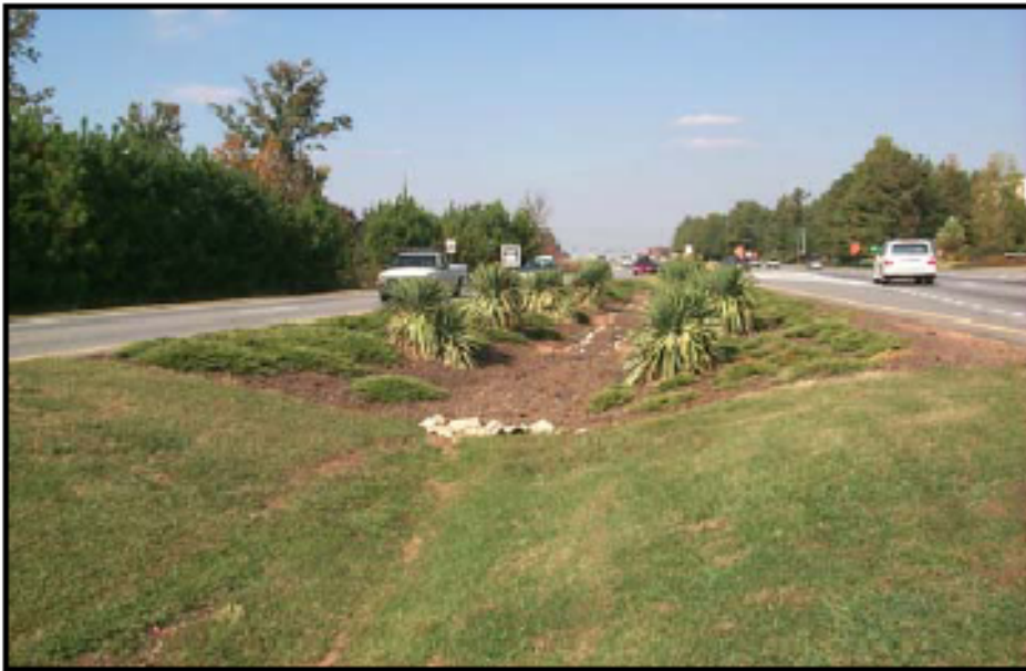
Enhanced Dry Swale ISWM Manual
