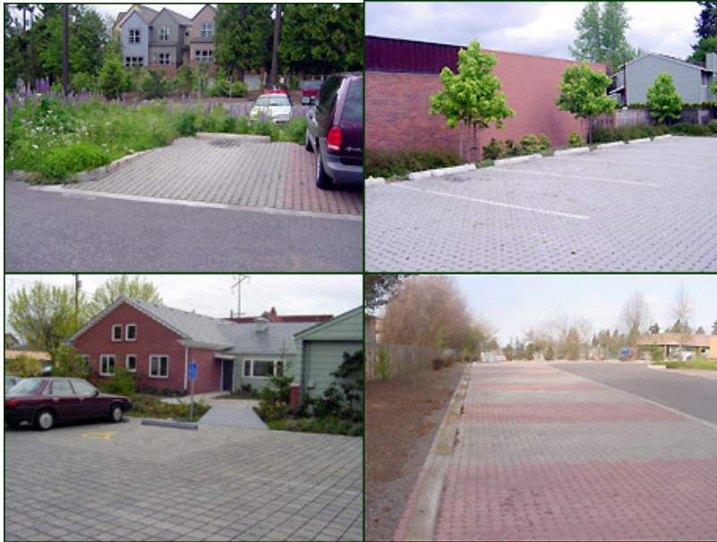
Examples of porous pavement uses for parking areas at office building and park facilities in Portland Oregon (Lower Columbia River Field Guide to Water Quality Friendly Development)
