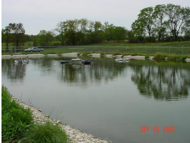
Polishing pond with SolarBee circulator (Photo from SolarBee Web site http://www.solarbee.com/picts.tpl )
