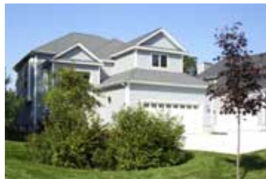
Rain garden bioretention cell for rooftop and driveway of single residence. (Massachusetts Low Impact Development Toolkit)
