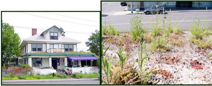
Example of green roof design at Peoples Food Coop, Portland, OR (Lower Columbia River Field Guide to Water Quality Friendly Development)
