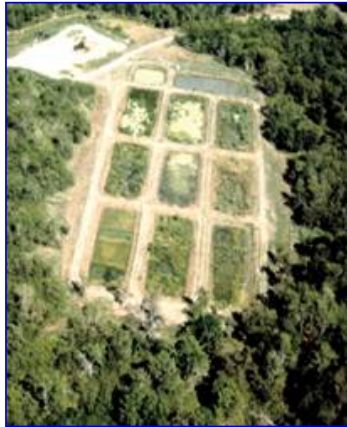
Tarrant Regional Water District's Pilot-Scale Demonstration Wetland (approximately 2.5 acres of wetland surface area) (Alan Plummer Associates Inc.)
