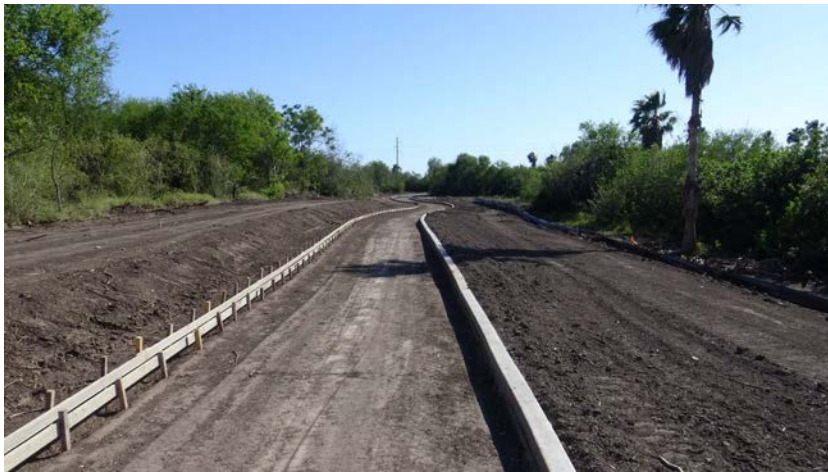
Heading east. Form and curb are visible.
