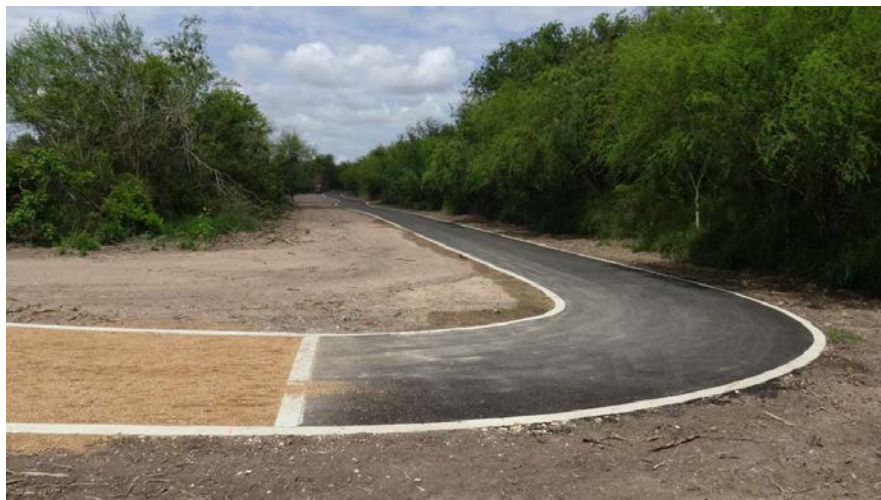
Looking back west from the east edge of the park property.
