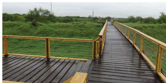
Refurbished piers in the San Benito Wetlands.
