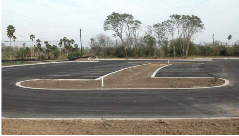
South end of the basin looking north toward the high school. Again, note the curves utilized in the design of the parking lot and basin.
