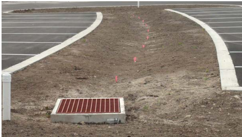
Bio-retention basin looking S.
