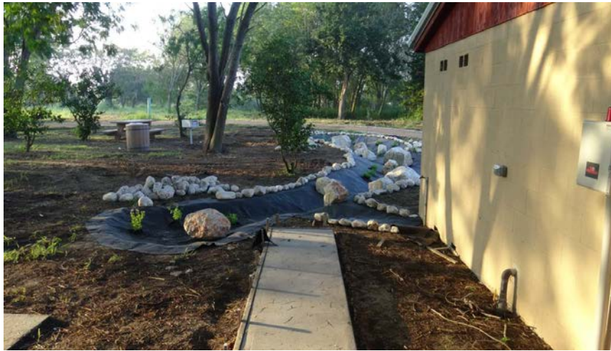
North end of pad looking south toward swale.
