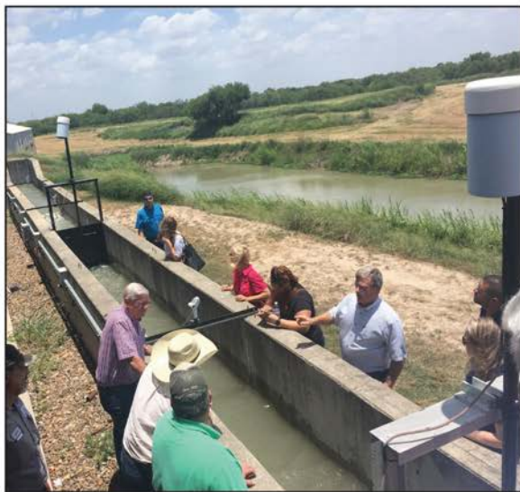
Tom McLemore, general manager, Harlingen Irrigation District, discusses the components and utility of the automated canal gate demonstration channel at the Rio Grande Center for Ag Water Efficiency.
