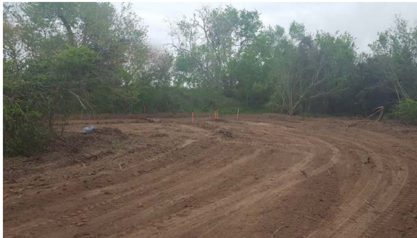
The U-turn looking north.
