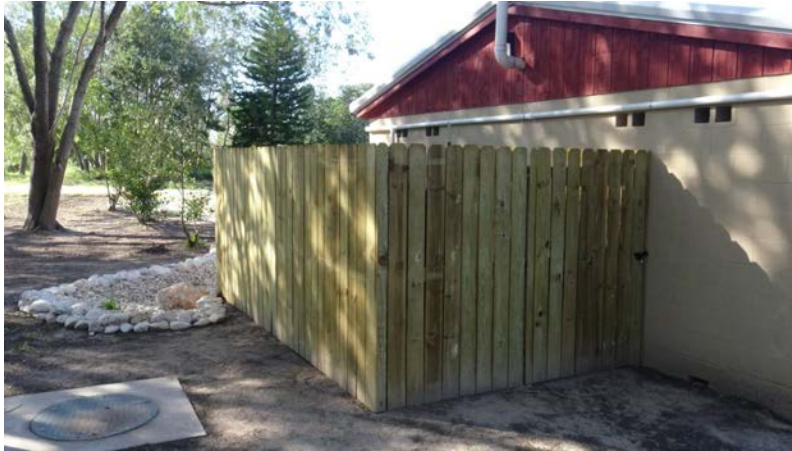
North end of privacy fence protecting rainwater harvesting collection system, looking south toward swale.
