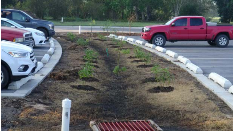
North end of the basin looking south, necklace pod-yellow sophora planted along the edge of basin.
