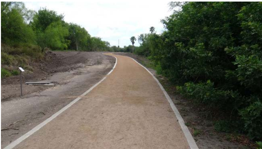
This is where the trail was joined to the newer section of the trail. You can see the difference in color of the crushed granite. Heading east.
