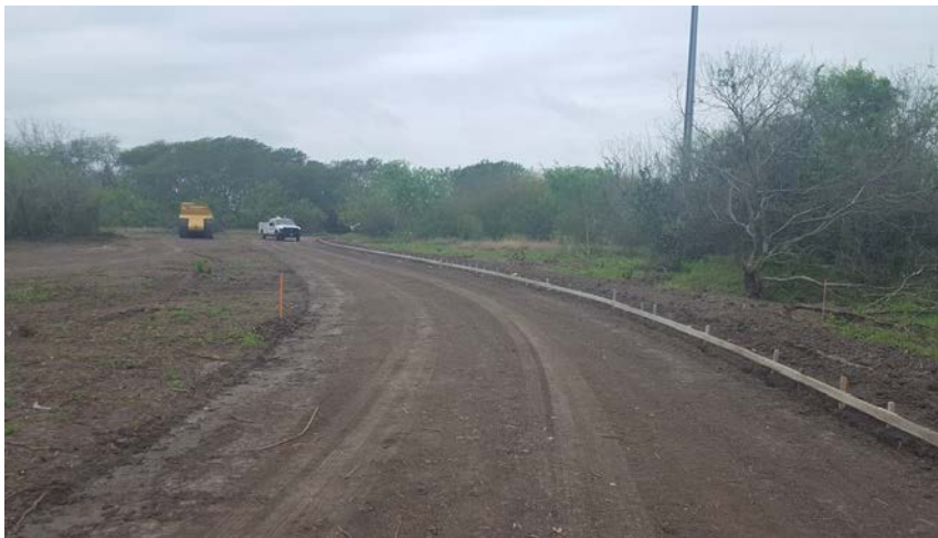
Heading west/southwest. Form for concrete is visible.
