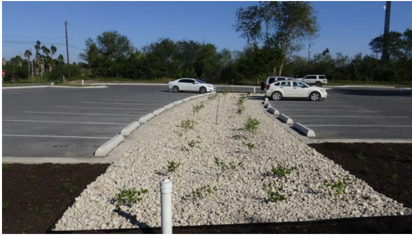
Mulch added to cover wild olive trees and gravel added to retention basin, south end of basin looking north.
