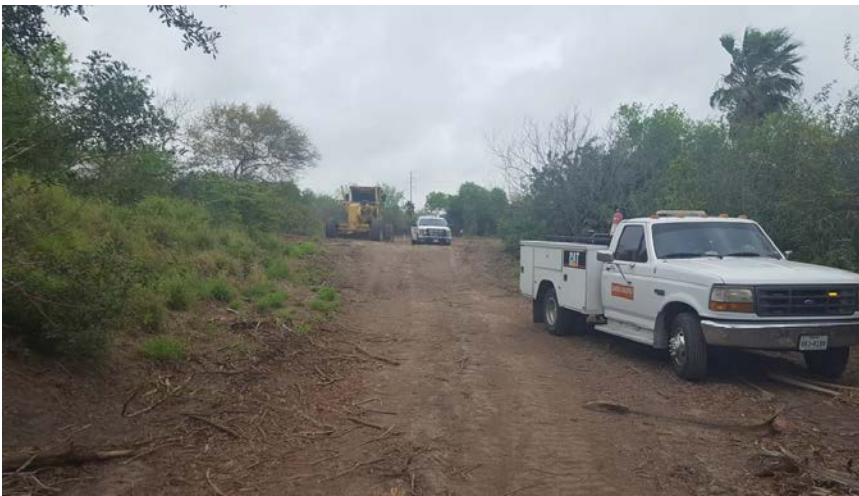
Looking back east. Maintainer is clearing vegetation for the trail.
