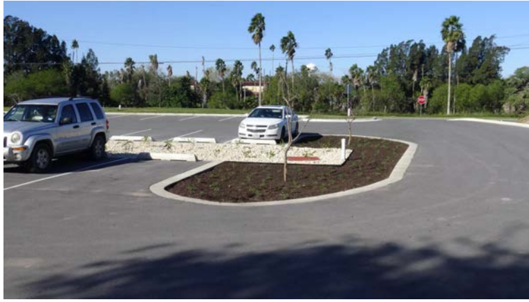
North end of bio-retention basin, standing east of the basin looking back to the west.
