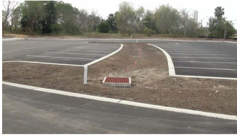
N end of the bio-retention basin looking S.
