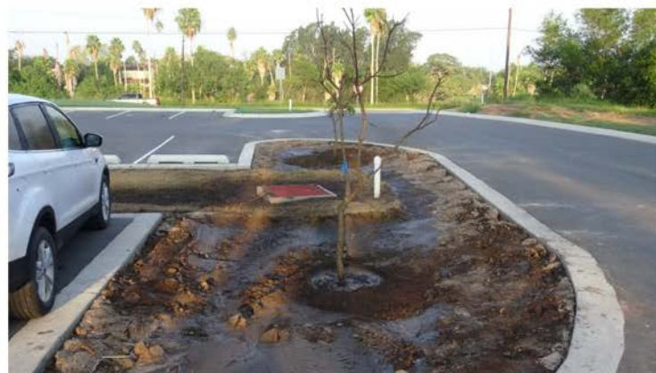
Wild olive trees planted in North section of basin looking west toward FM 1847.
