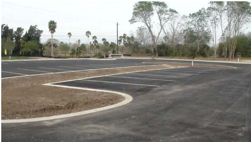
South end of the basin looking northwest toward entrance and FM 1847.
