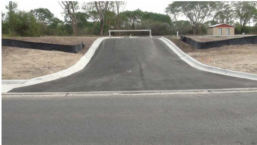
Entrance to the Los Fresnos Nature Park, looking east off of FM 1847. Note the elevation difference between FM 1847 and the parking lot and the silt fencing around the construction areas.
