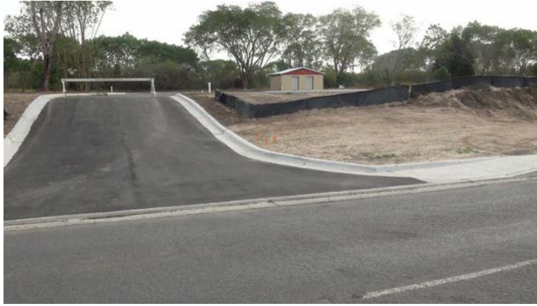
Entrance looking SE.
