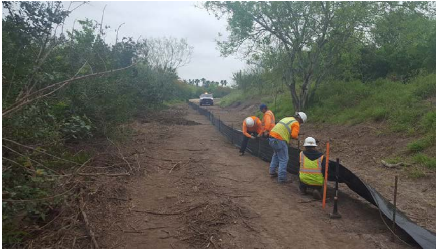
Looking back toward the west and Phase I of the trail.
