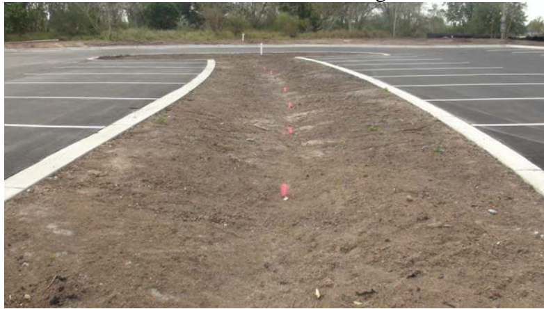
Close up view of the slope in the bio-retention basin.
