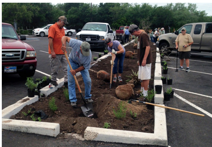
A bio-retention basin was built at Ramsey Park and planted with native plants and trees.
