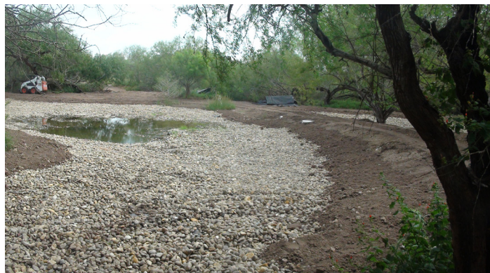
The bio-retention basin at Ramsey Park filters stormwater runoff from the parking lot into a newly expanded wetland area in the park.
