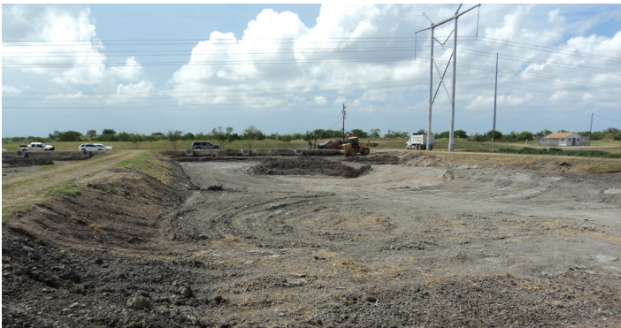
Clearing and leveling is undertaken in one of the San Benito wetland cells before filling with water.
