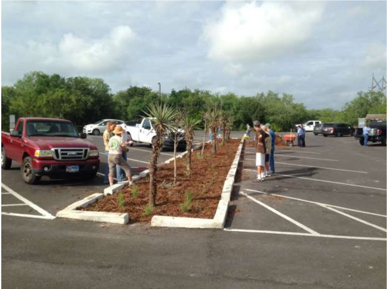
Planting of the Bio-retention Basin complete.
