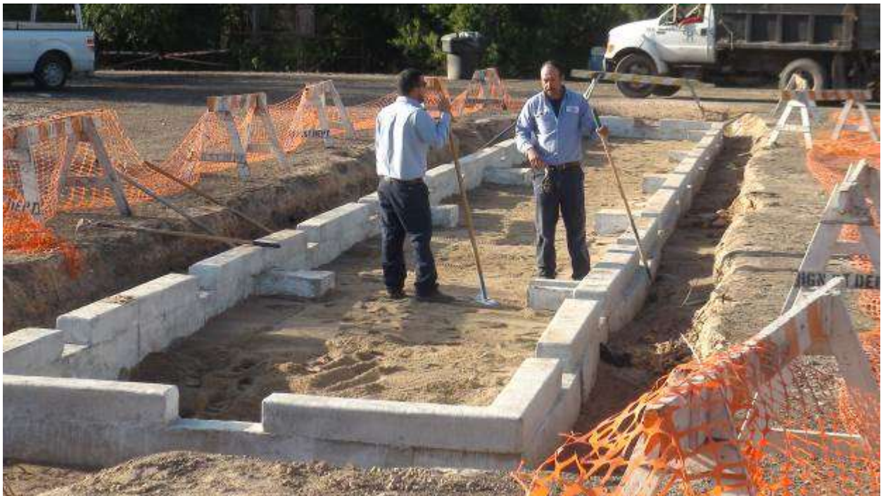
COH filling bio-retention basin with sand layer.
