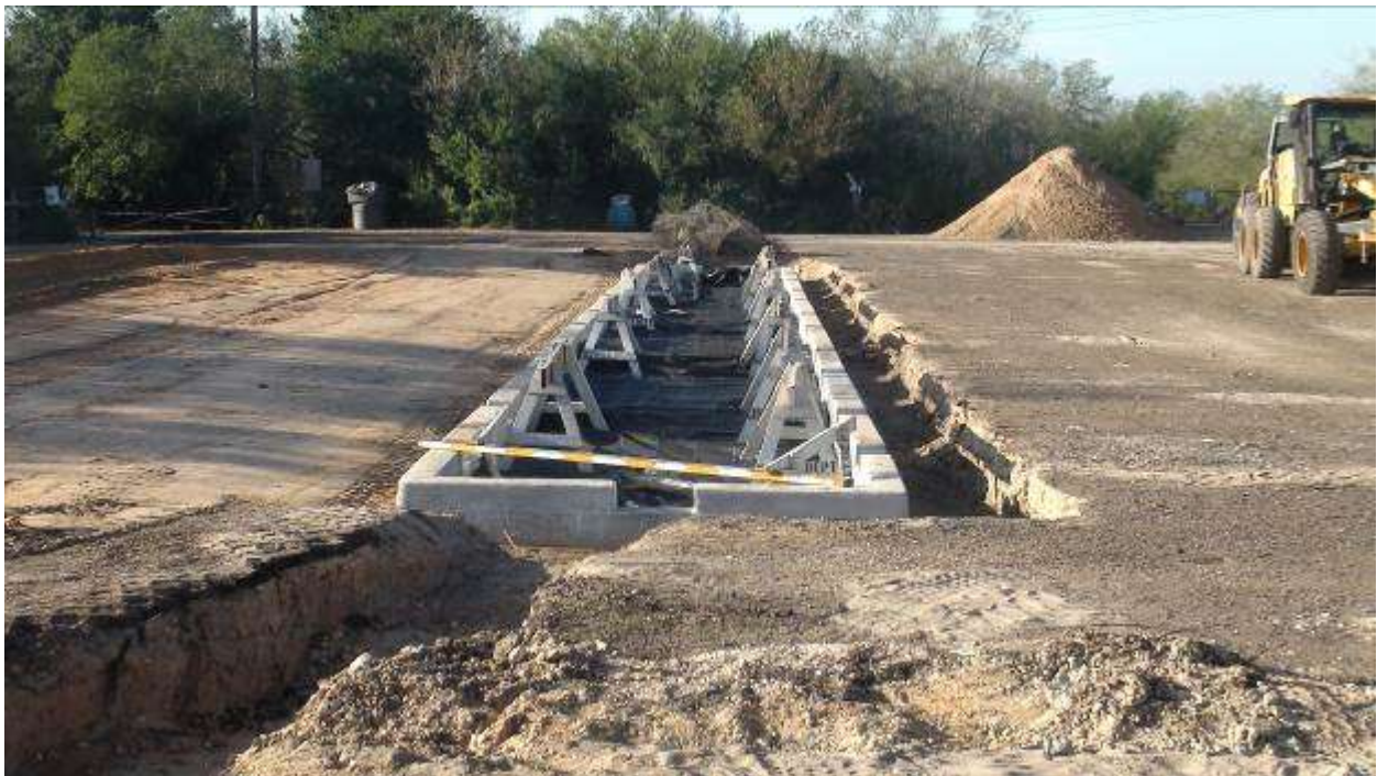
Bio-retention basin awaiting top soil and plant material
