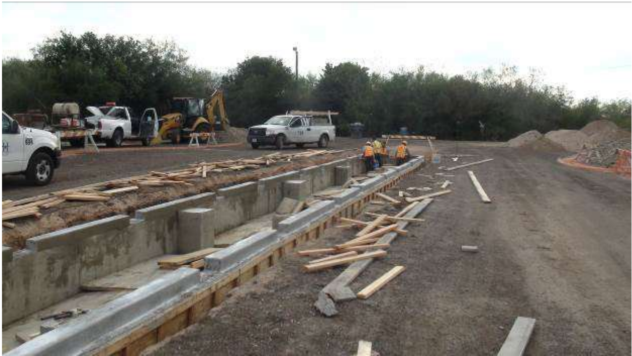
Construction of Bio-retention complete.
