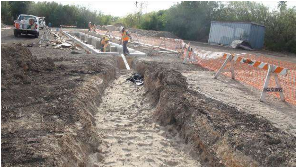
COH crew backfilling trench for discharge pipe.
