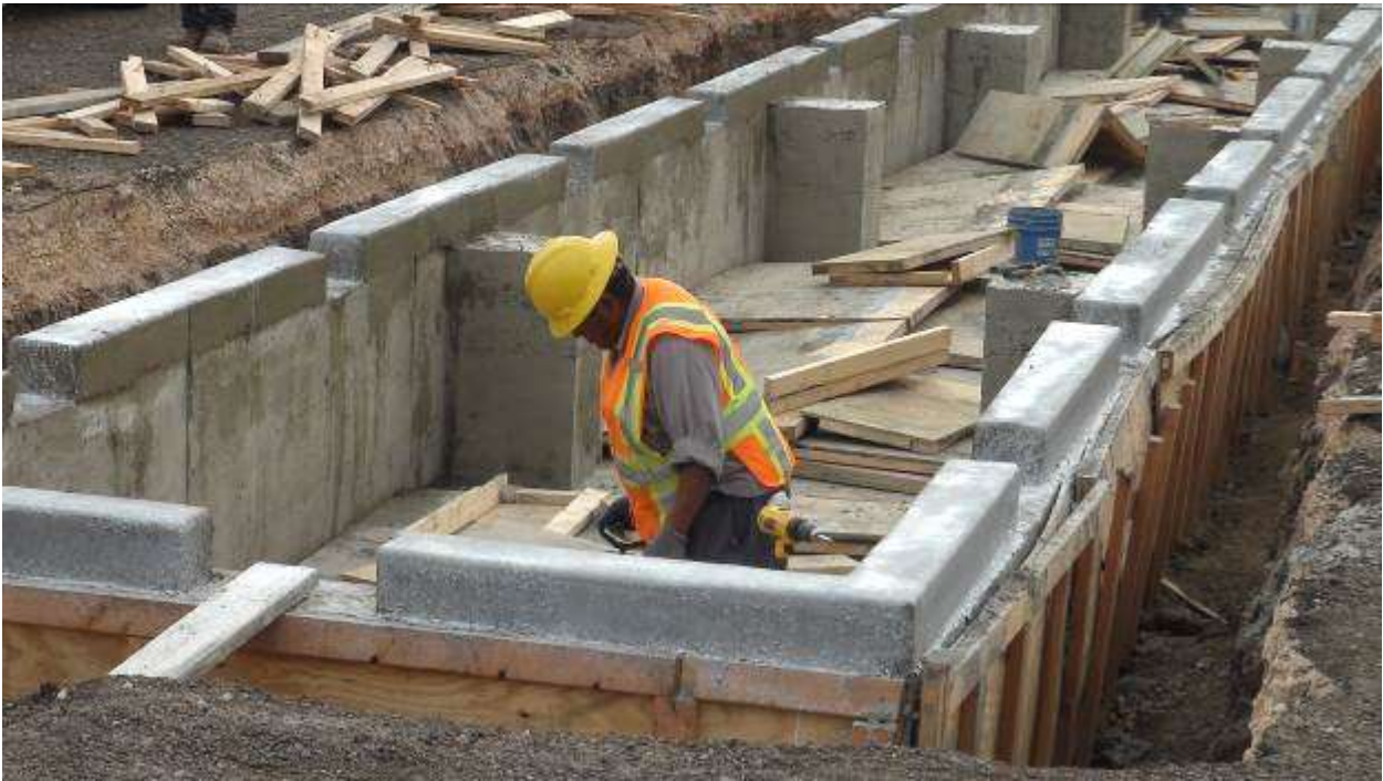
Removing the forms from the wall the concrete has cured.
