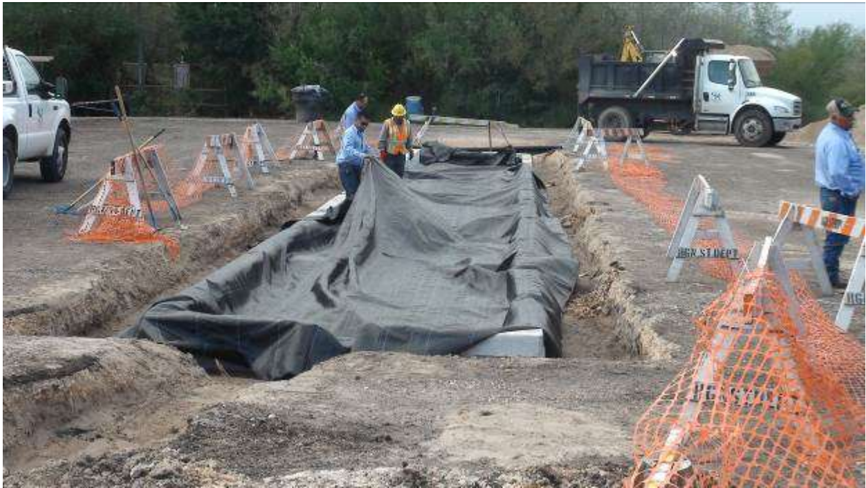
COH crew placing landscaping fabric over sand layer.
